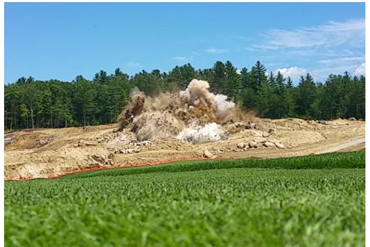
Demolition of ledge rock on the new #18
