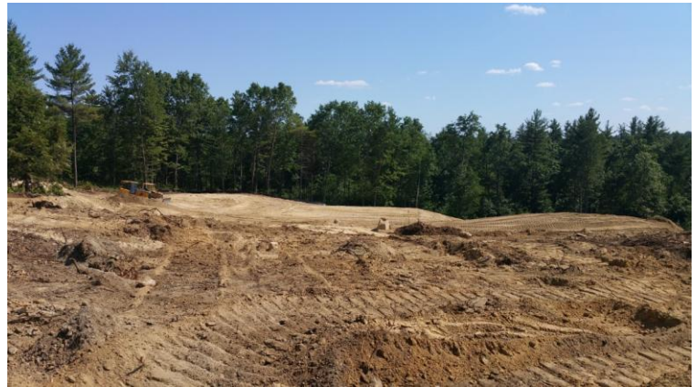
New 10 th tee complex being constructed
