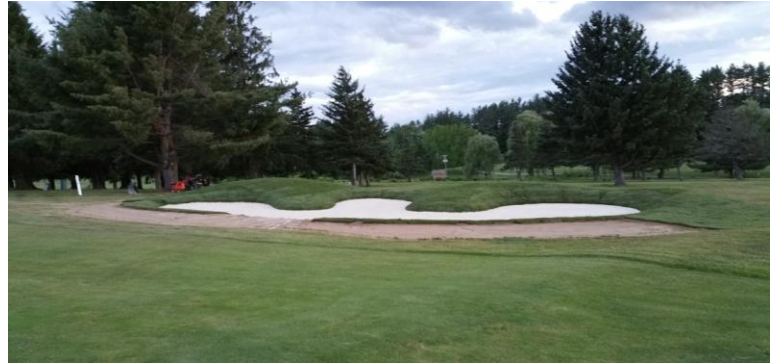
New fairway bunker being constructed on hole #5
